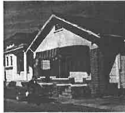
Porch that reduces heat gain from sun.
