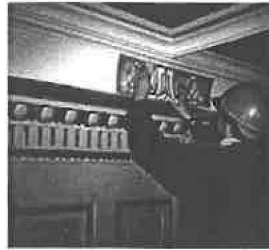
Painted interior finishes repaired during rehabilitation.
