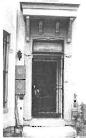
Inappropriate installation of new meters on primary elevation.
