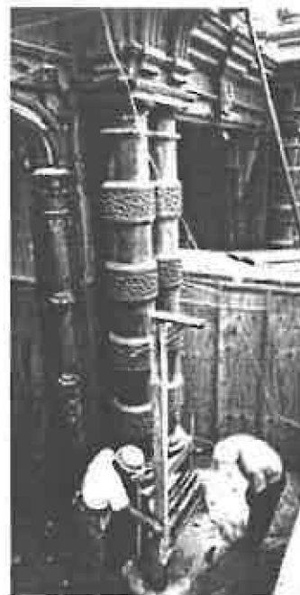
Missing cast-iron elements replaced with cast aluminum.
