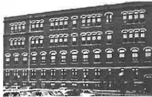
Distinctive window design on 19th century building.
