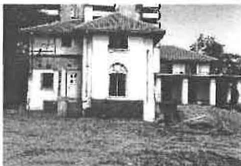
Important site features destroyed during rehabilitation.
