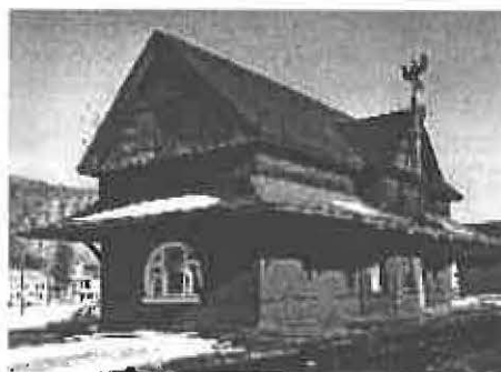
Gable and pent roof in excellent condition.
