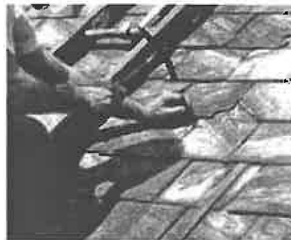
Repairing slate roof using traditional methods.
