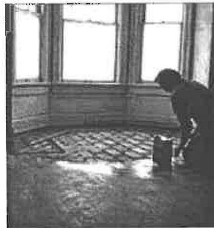
Applying a protective finish to historic flooring.
