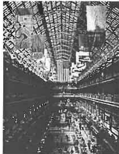
Historic shopping arcade following successful rehabilitation.
