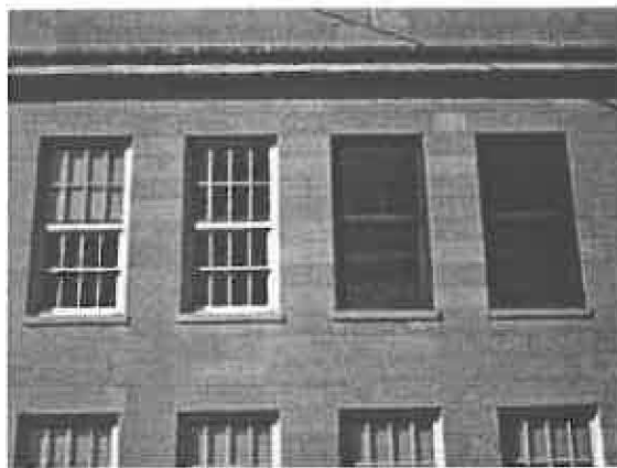
Historic windows (left) on primary elevation inappropriately replaced with tinted glazing (right). Photo: Mike Jackson.
