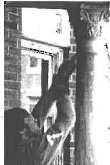
Hand scraping wood column prior to repainting.
