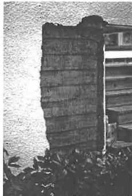
Preparation for stucco repair.
