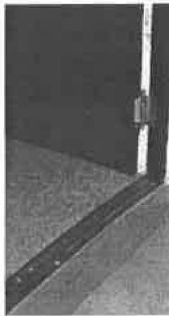
Historic threshold made accessible with 1/2" wood bevel.
