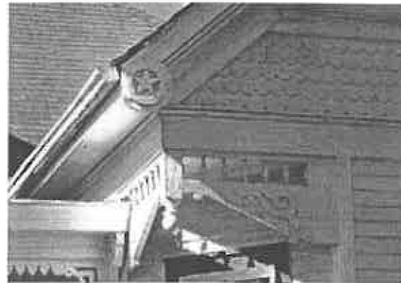
Decorative exterior wood trim and siding.
