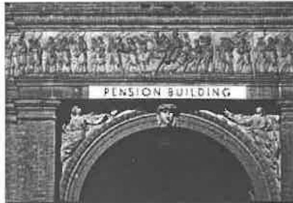
1880s brick building with terracotta trim.
