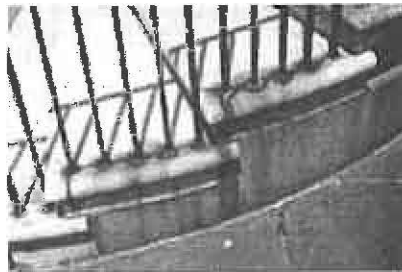
Chemical reaction between new concrete steps and historic iron railing that causes unsightly appearance.
