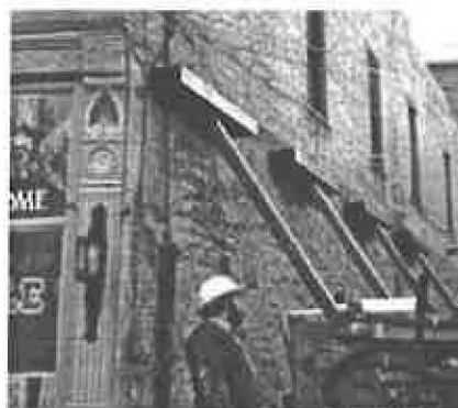
Structural stabilization of masonry walls before rehabilitation.
