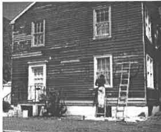
Limited replacement in-kind of deteriorated wood clapboards.
