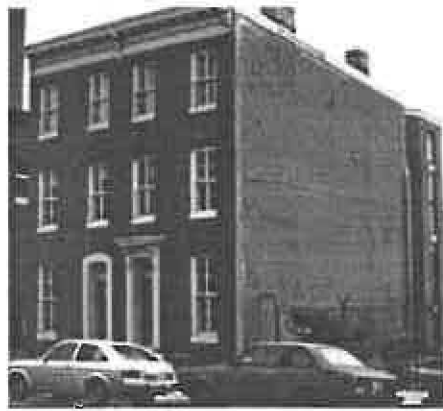
Small, compatible stairtower on rear elevation.
