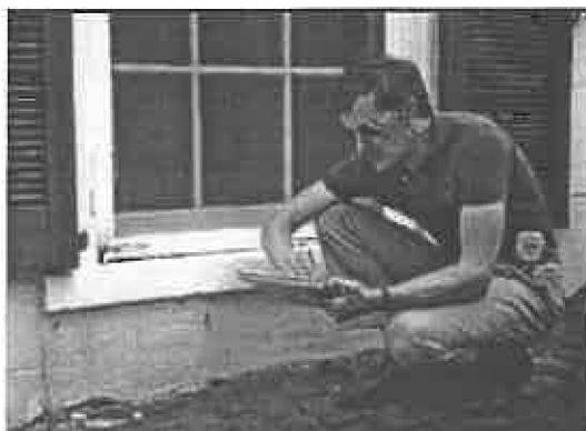
Window condition assessment preceding repair work.
