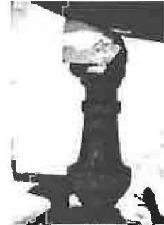
Surviving baluster of terrace that provides a prototype to replace damaged balusters.
