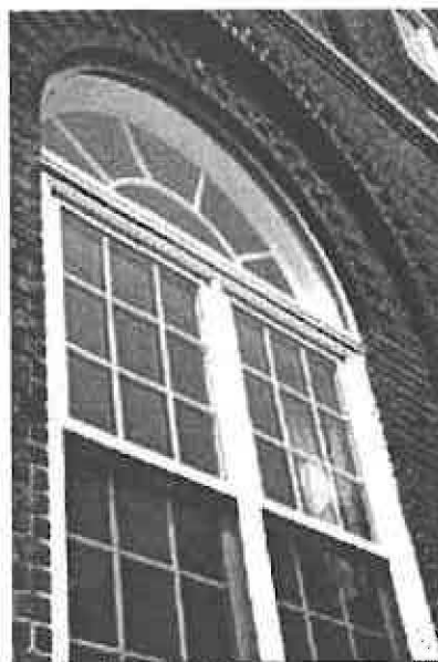
Newly painted double-hung wood windows.
