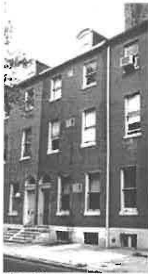
Historic building material destroyed by through-the-wall air-conditioners.
