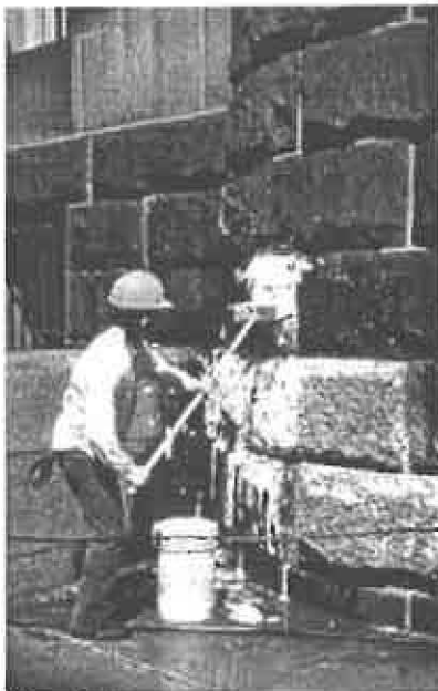
Chemical cleaning to remove dirt from granite.
